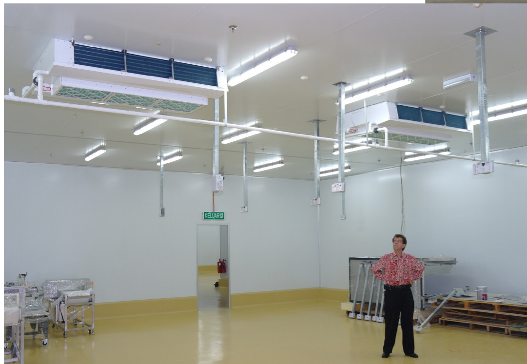
Dual air discharge units. 16 °C Processing room
