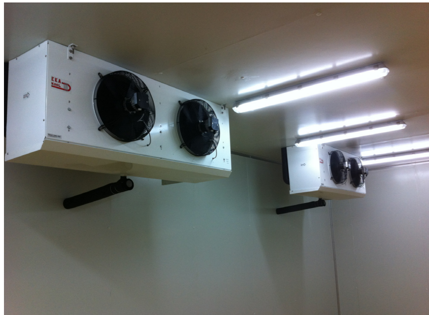
-20 °C and +3 °C, Dual Purpose storage room
