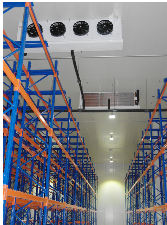
-20 °C Cold room
